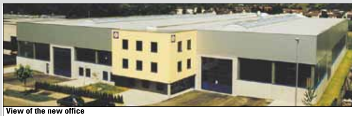
View of the new office
