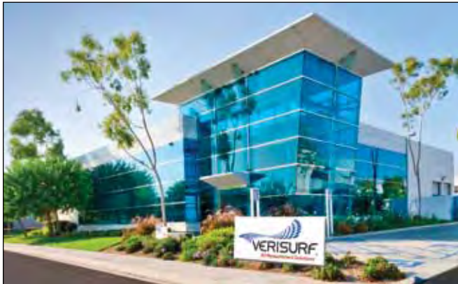
Verisurf expanded into a new corporate headquarters located in Anaheim, California (courtesy of Verisurf Software).
