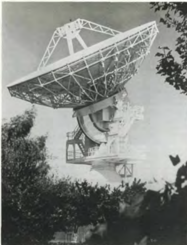
Fig. 8—Microwave antenna with az-el mount.
