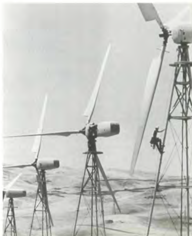
Fig. 2 - Wind turbine generators.
