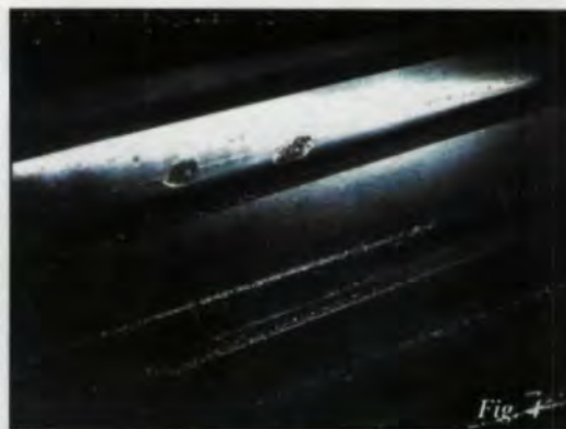
Fig. 4—Pitting distress on second mill pinion teeth.
