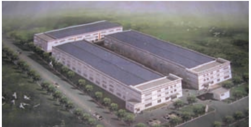
The just-opened, 22,600-sq. ft. Gleason Gear Technology (Suzhou) Co. Ltd., which will produce machine tools and possibly other products exclusively for the Chinese market.
