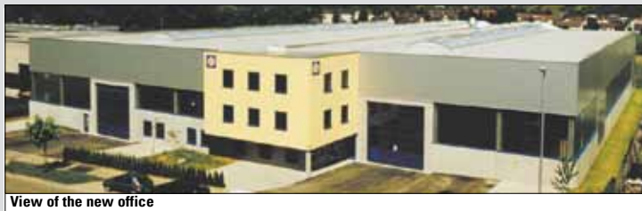
View of the new office
