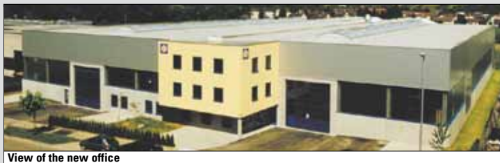
View of the new office
