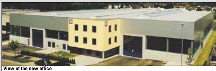
View of the new office
