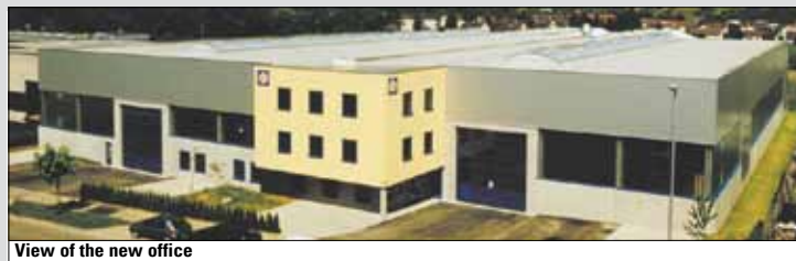
View of the new office
