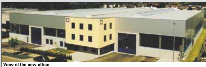
View of the new office
