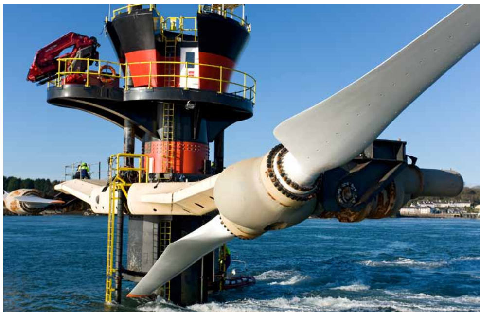
The SeaGen power plant is located in a strait in the natural harbor Strangford Lough. The turbine is attached to a pile structure swept by the tidal currents, which is anchored to the seabed at a depth of approximately 30 meters. The turbine's rotor blades are driven by the water currents (courtesy of Siemens).
