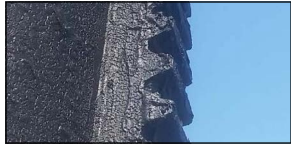
Figure 20 Greased rack for operation.
