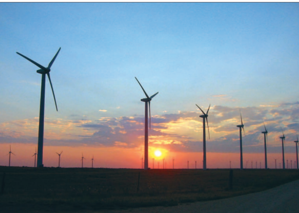
Wind turbines spanning the horizon bear testament to successful efforts by Iowa's governor and legislature to attract industry-related OEMs and suppliers to their state. The benefits are two-fold: clean alternative energy and well-paying jobs. Photo courtesy of Mitsubishi.
