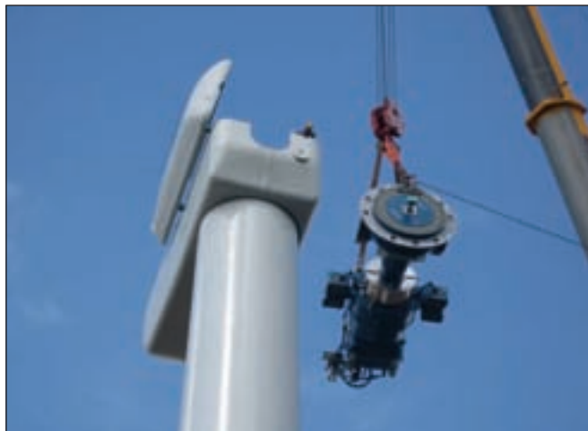
Hoisting a drivetrain up to its nacelle home. Courtesy Paul Anderson.
