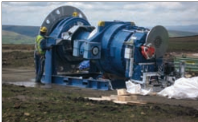
A worker prepares the drivetrain for installation. Courtesy Paul Anderson.
