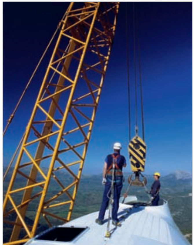
Workers constructing a wind turbine in Didima, Greece. Courtesy Vestas.
