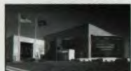
Schafer Gear Works, Inc.
