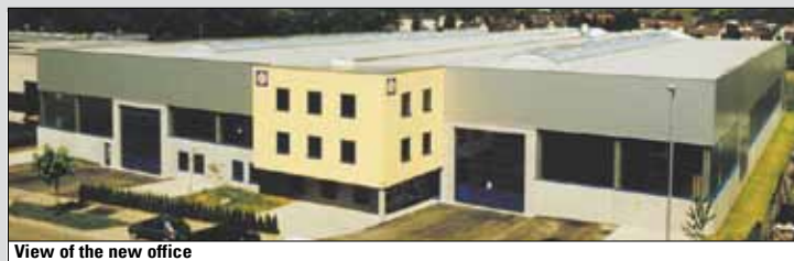
View of the new office
