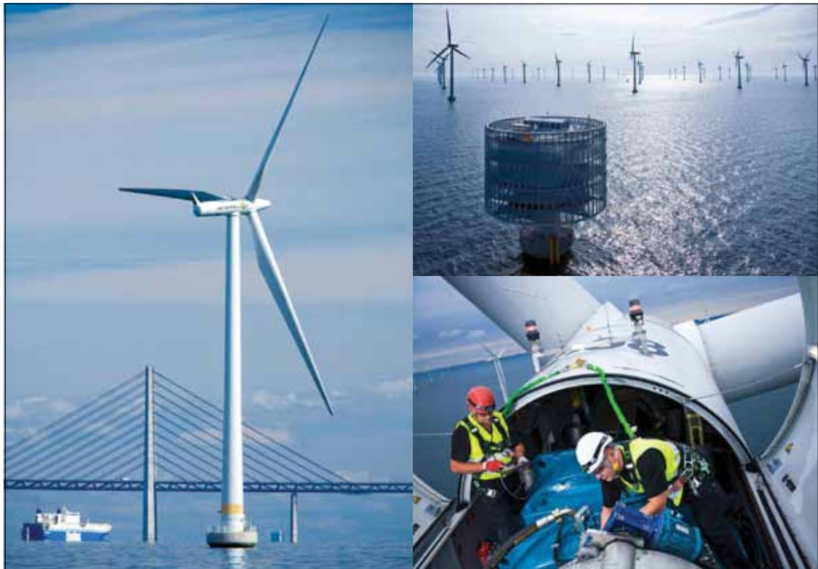
Gear science and manufacturing technology will play a key role in wind power technology's continued evolution and widespread acceptance. (Photos this page courtesy Siemens Corp.)
