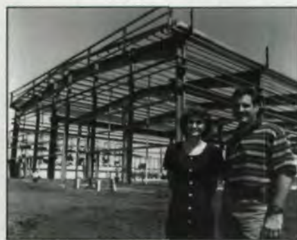
Advanced Heat Treat's expansion project.
