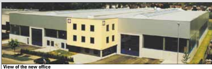
View of the new office
