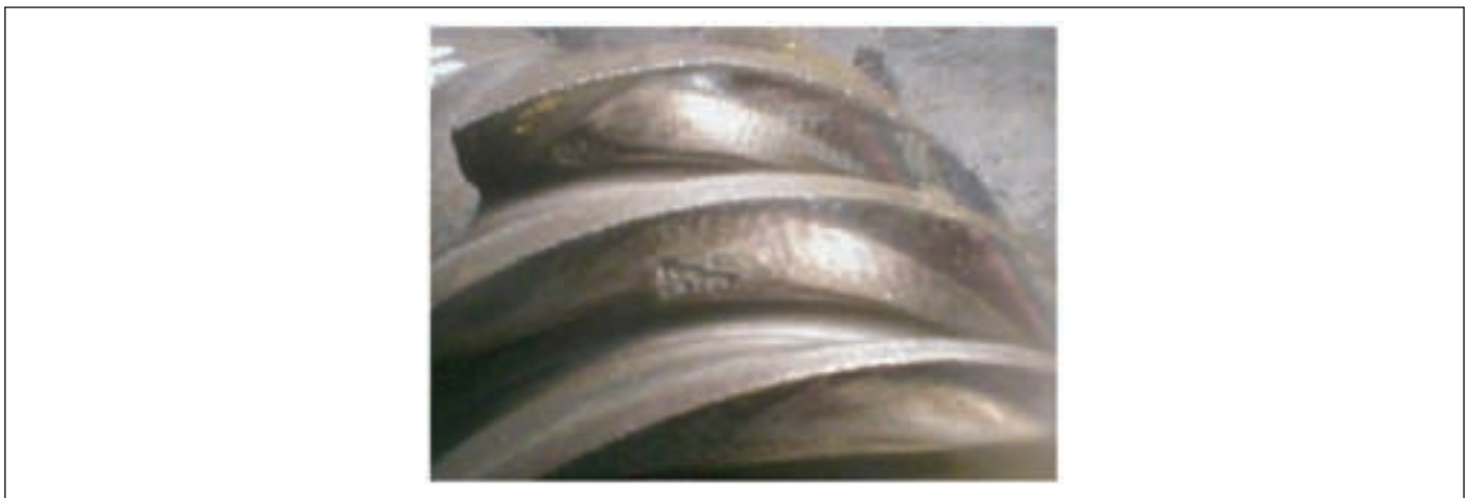
Figure 14—Representative pinion failures of the seven test samples.
