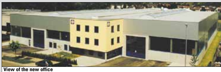
View of the new office
