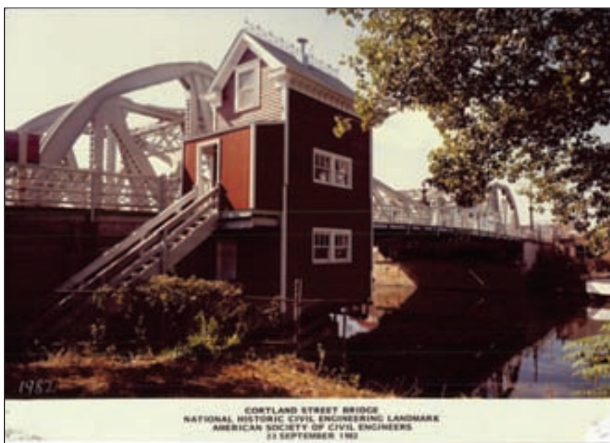
Cortland Street Bridge—the first movable bridge built in Chicago (1902) and a national historic civil engineering landmark. (Photo courtesy of City of Chicago)
