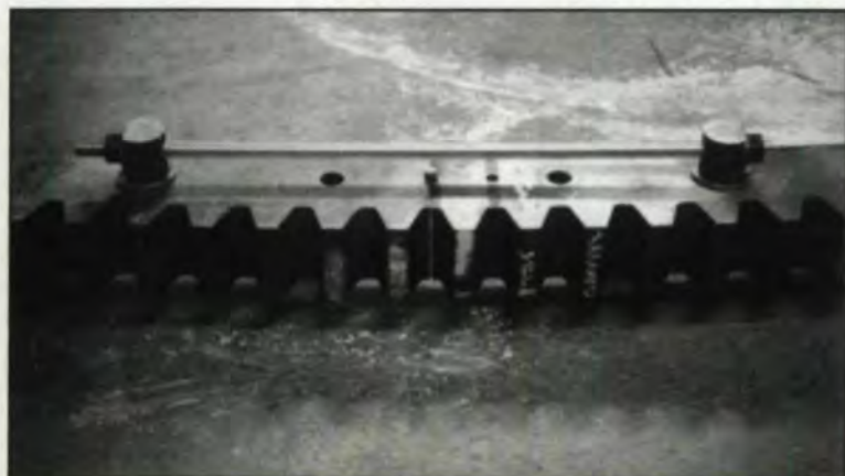
Fig. 1 — A close up view of the gear shows how the toothed sections were assembled during the roundup. Sections had to fit together with a very tight tolerance of \pm 5 mm on the 62' diameter.
