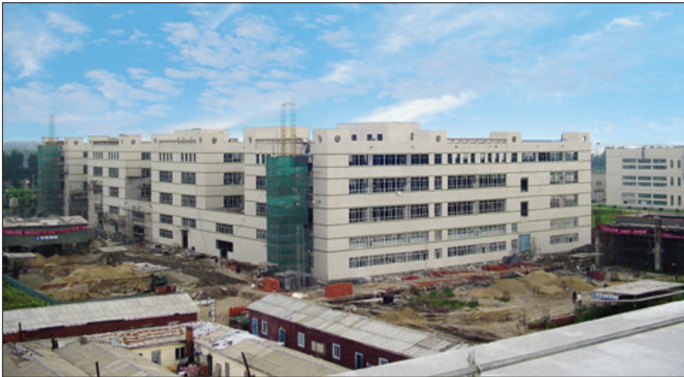
Gleason built a factory in Harbin, China to be closer to its customers.
