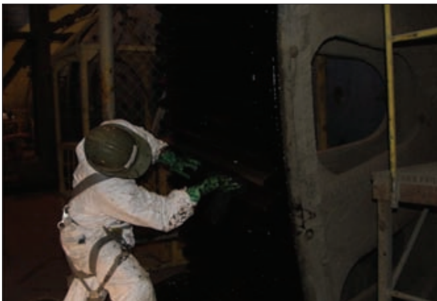
Drago examines a SAG mill gear, which is about 35 feet in diameter, at a copper mine in Chile in order to determine the cause of tooth surface fatigue damage.
