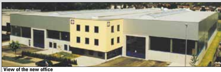
View of the new office
