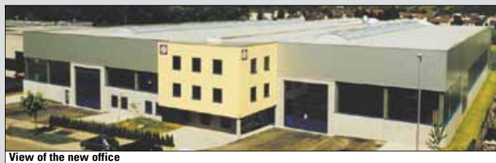
View of the new office
