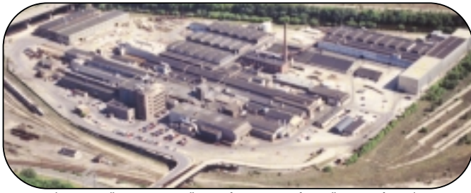
Flying Over Falk—In America, Falk's main factory consists of 1.1 million square feet and is the bulk of Falk's worldwide manufacturing space, about 1.8 million square feet.
