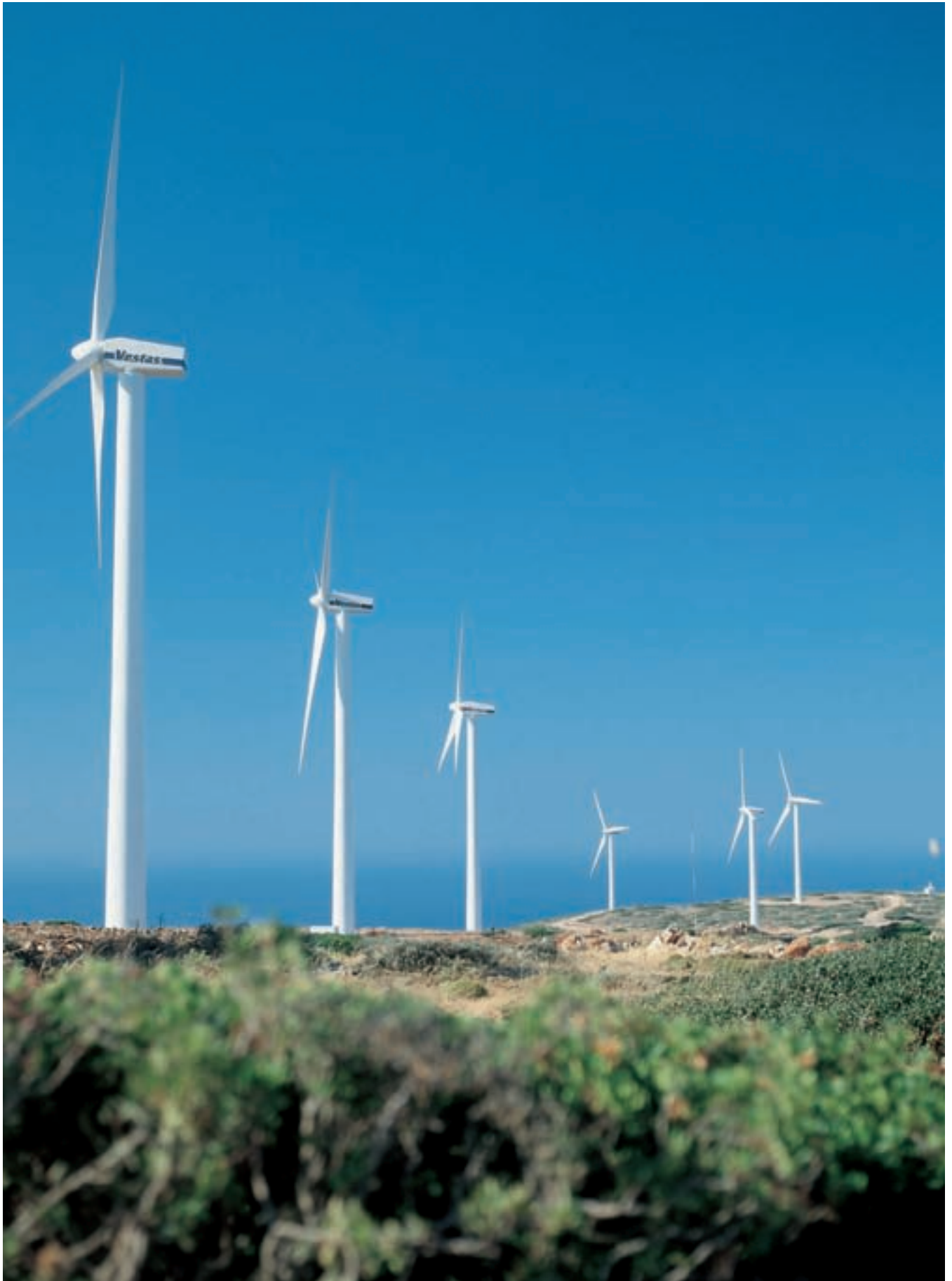
A bumper crop in wind farming will continue in 2009, especially with the recent extension of the energy tax credit by Congress. (Photo courtesy of Vestas.)
